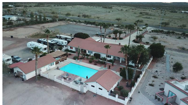
Main Building (above the pool)
